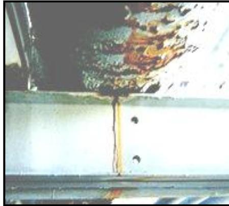
Corrosion at Pipe support locations leading to leaks
