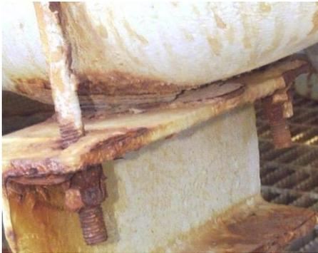
Corrosion at Pipe support locations
